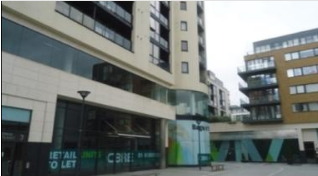
Plate 1: Chamber Square with an unused building (foreground) and a formally used unit (background)
