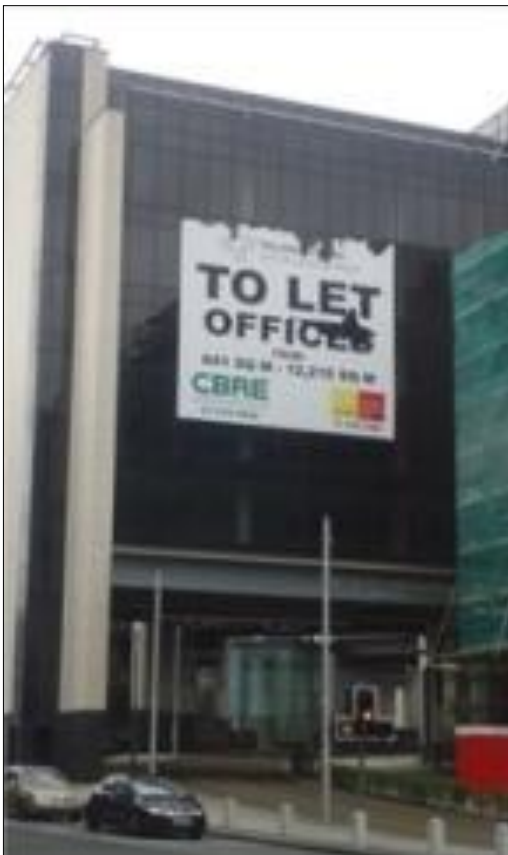
Plate 2: Tallaght Cross West, unused office building
